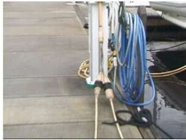
Figure 2. This is a power pedestal on a dock that supplies electric power (shore power) to a boat. A single 50 amp 220vAC shore power cord (light yellow) splits into two (2) 30 amp 110 VAC feeds. This item is known as a "Y adapter" and commonly used for boats that have two (2) 30 amp 120 VAC inlets. There is electrical resistance building up on the left leg of the "Y adapter" and it should be scheduled to be replaced.
